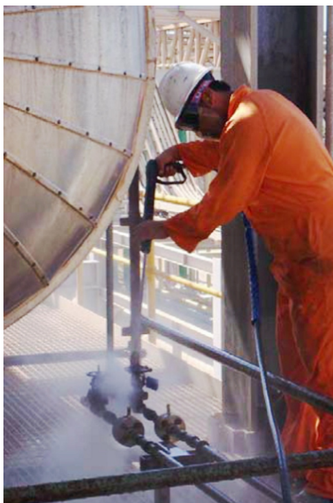
Below: pressure washing to remove heavy grease.
