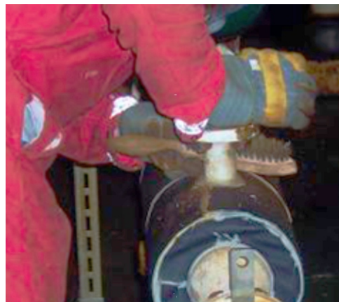
Above: surface preparation using wire brush on flange.
