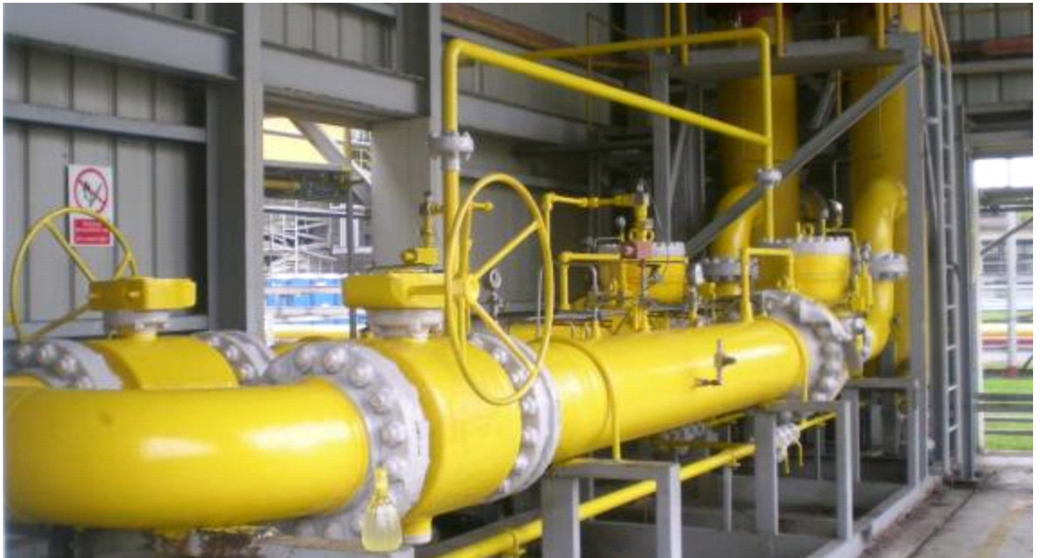
Above right and below: pipelines coated in Alocit with the addition of Enviropeel on bolted areas to provide the best possible protection.
