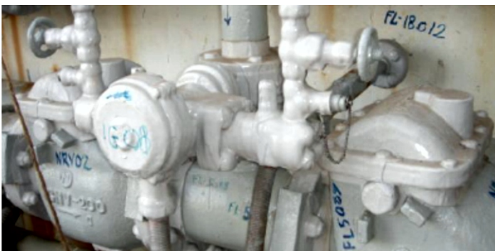
Top: spraying Enviropeel on a flange joint Above: protected flanges on an LPG carrier Right: Enviropeel protection on a conveyor bearing and shaft
