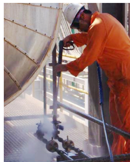
Above: surface preparation using wire brush. Below: pressure washing to remove heavy grease.
