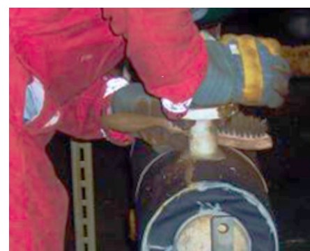
Above: surface preparation using wire brush. Below: pressure washing to remove heavy grease.
