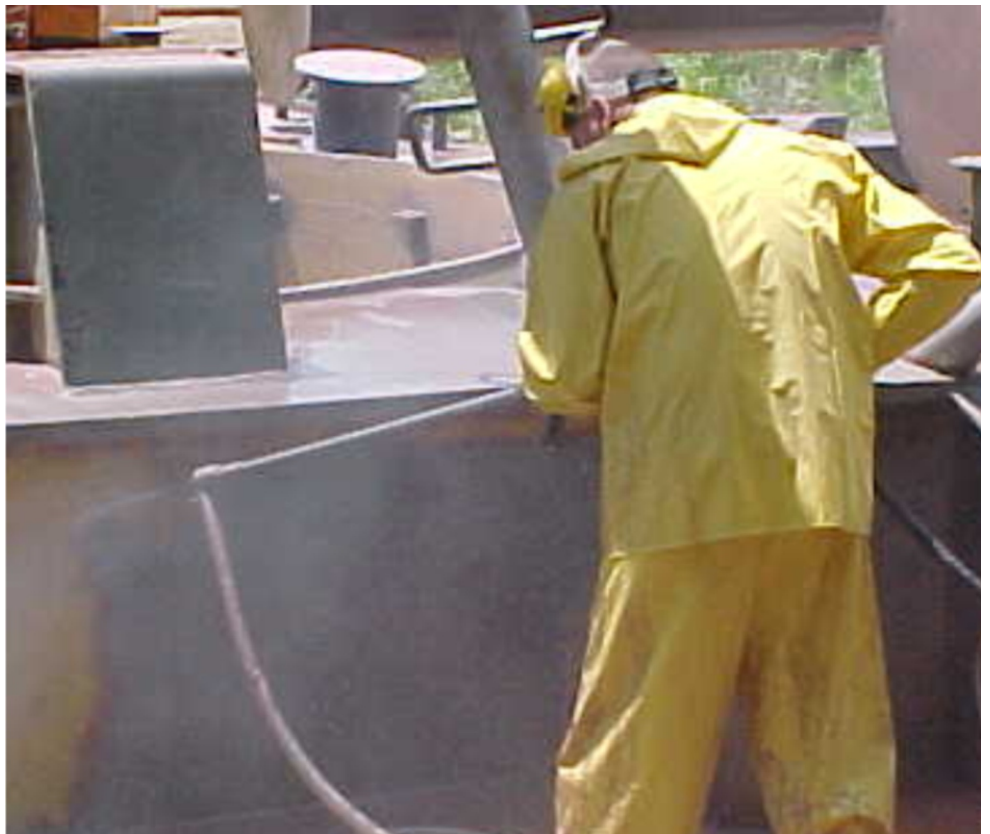
Above: Water-jetting is a fast and clean surface preparation method. Using blast media with the water gave profile, the ability to use Alocit immediately after cleaning while still wet achieved significant cost savings.
