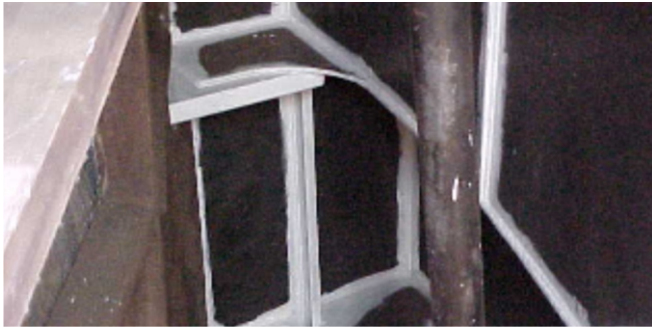
Above: Inside the coffer dams after coating Above left: Buoy bottom after water-jetting Left: Stripe coating cofferdam with 28.15
