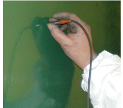
Below: testing the finished coating, results shown in panel below
