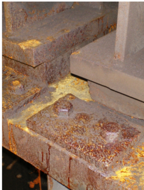
Top: the rail bridge was severely affected by the freezing conditions Above left: the condition of the blasted substrate awaiting coating Above right: manually applying the test coating to a freezing, wet substrate Below: spray-applying the first coat of Alocit
