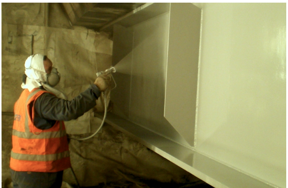
Top: the rail bridge was severely affected by the freezing conditions Above left: the condition of the blasted substrate awaiting coating Above right: manually applying the test coating to a freezing, wet substrate Below: spray-applying the first coat of Alocit
