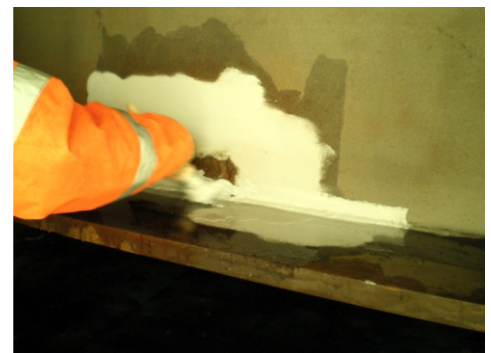
Top: the rail bridge was severely affected by the freezing conditions Above left: the condition of the blasted substrate awaiting coating Above right: manually applying the test coating to a freezing, wet substrate Below: spray-applying the first coat of Alocit
