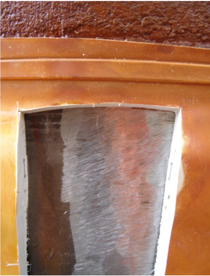
Fig.9 above: the removal of the mill scale is clearly visible
