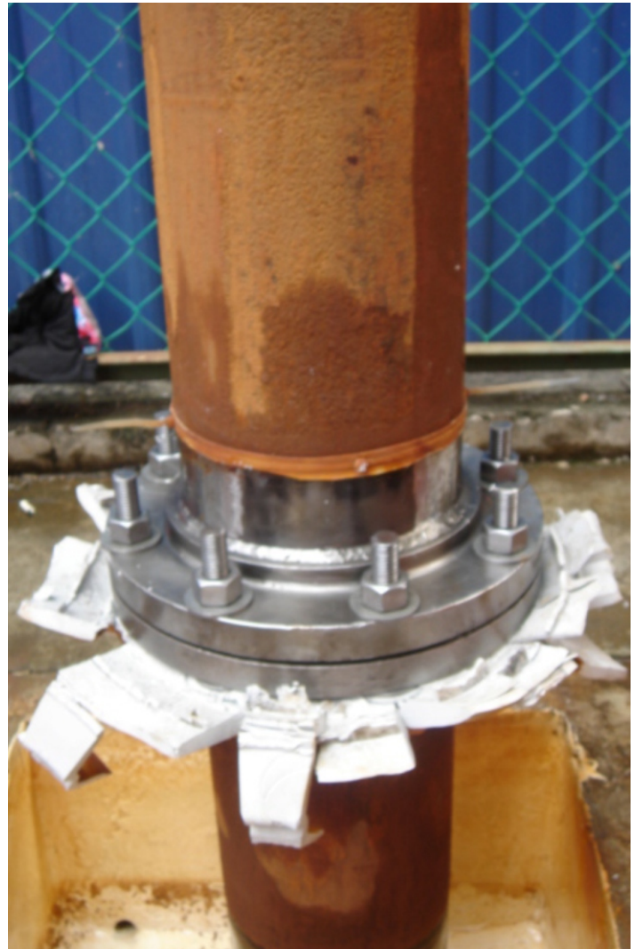
Fig.10 above right: following removal of all the Enviropeel material from the joint, the level of protection is clearly visible - no rust or staining to be seen.
