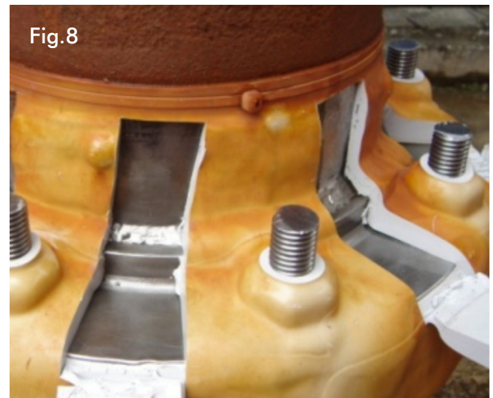
Fig.8 bottom right: strips of Enviropeel have been removed to reveal the substrate below.
