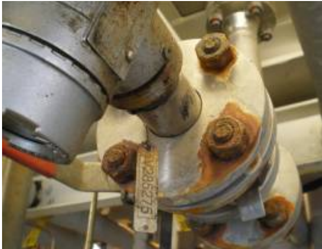
Figures 2 and 3: zinc-nickel plated L7 bolts on stainless steel flanges
