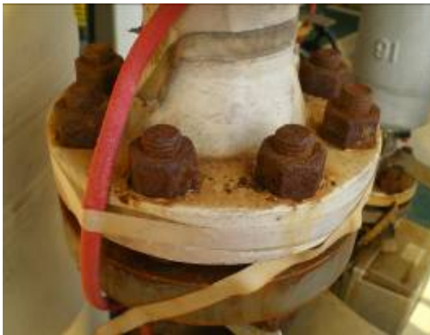
Figures 4 and 5: zinc-nickel plated L7 bolts on a mixed stainless/carbon steel substrate
